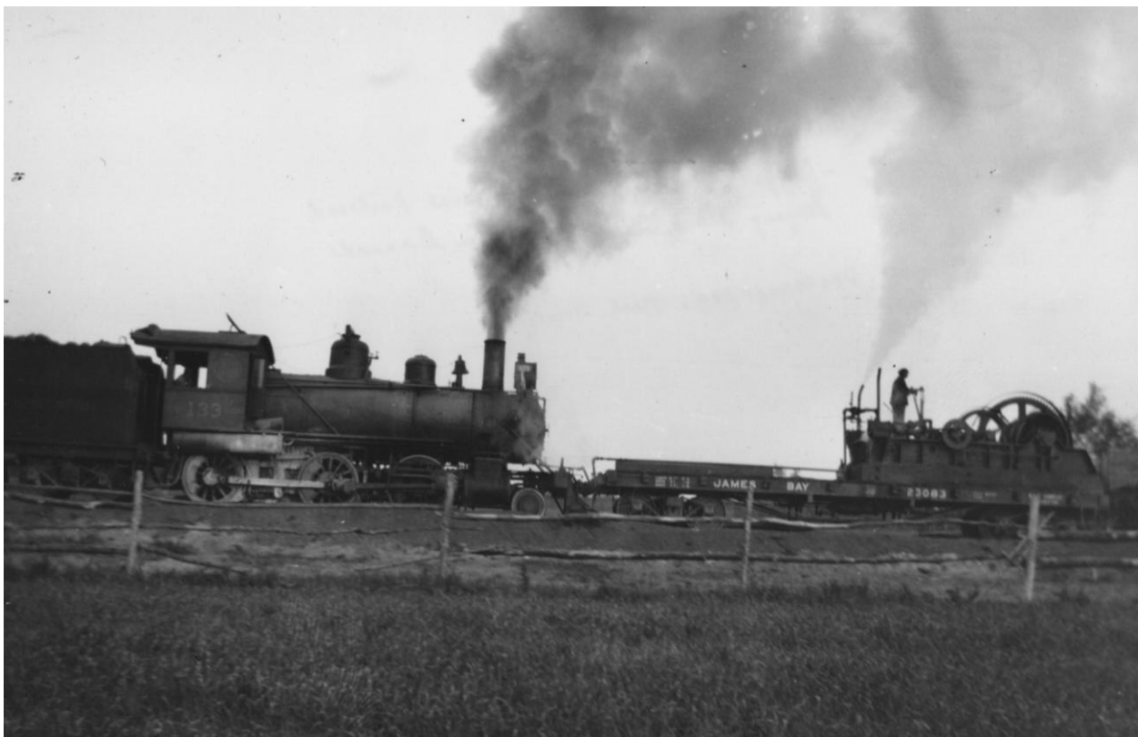
Locomotive #133, July 1914, laying tracks north of Fisher Branch, Manitoba
